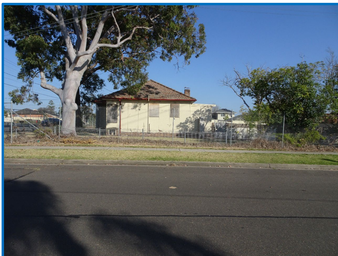
Figure 3c: Photograph of the Site frontage on Stimson Street
